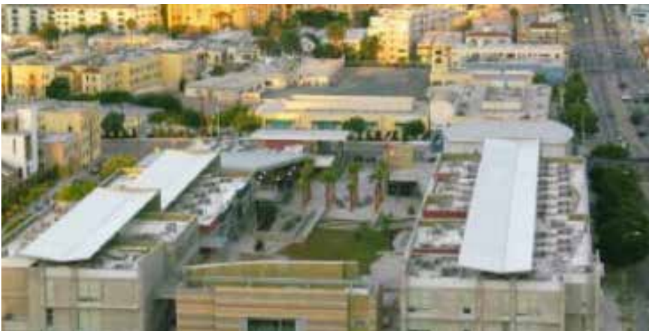
New Deck installed on the unused roof of a Los Angeles Unified High School. The roof was re-tasked as a partial green roof with food service and commons.
